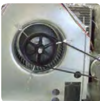
PowerMax DriveN Pulley on a Centrifugal Fan.
